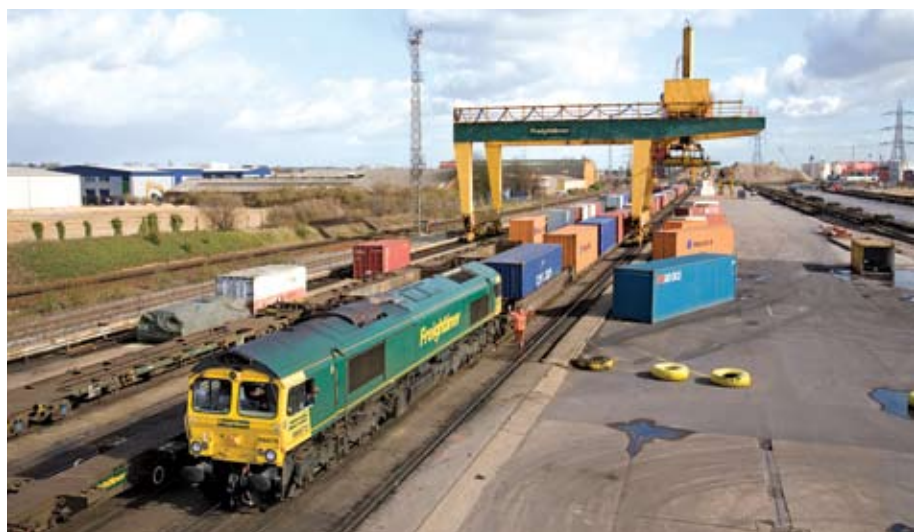
Intermodal container operations are underway at Freightliner's Southampton Maritime terminal which serves the second largest port for deep sea rail traffic in the UK. Network RUS forecasts predict that demand for this type of service will grow by up to 300% in the period to the mid-2030s. Gordon White
